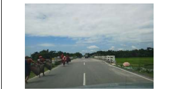
Fig. 12. Chainage – 7/130 Km (Minor Bridge)
